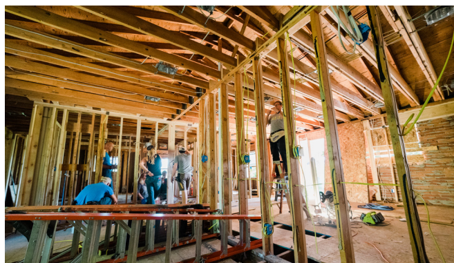
Volunteers from Covenant OPC in Sinking Spring, PA, New Hope Presbyterian in Bridgeton, NJ, and Redeemer Presbyterian in Ada, MI, work on rewiring
