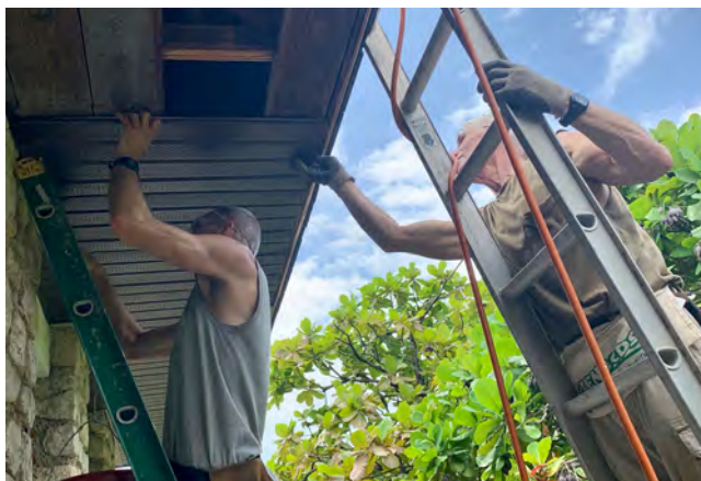
Installing rest soffits to prepare for the Kaliko roof project
