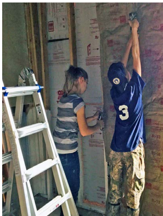
Laura Harness and Dick Boermann stapling insulation
