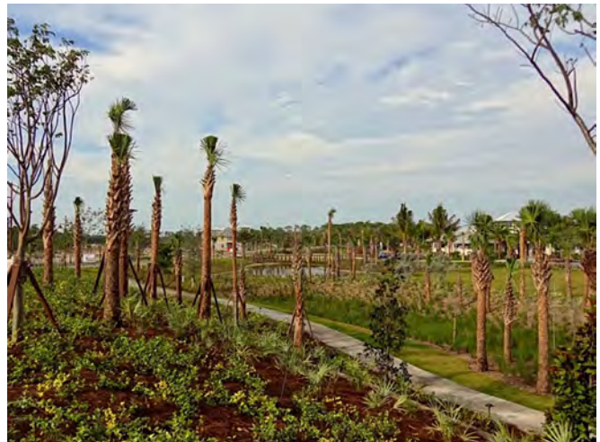
A large gated community under construction in Naples
